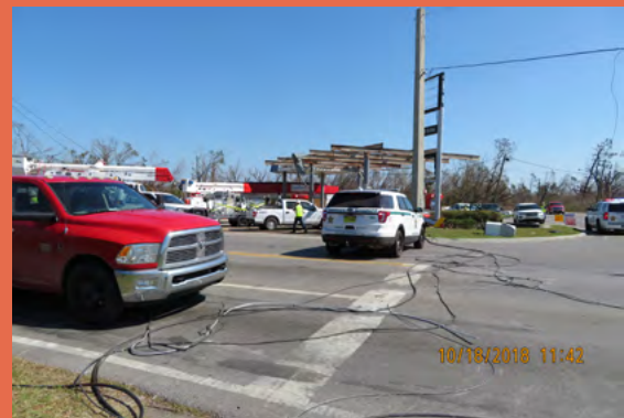
ABOVE An intersection in Bay County showing fallen power lines and crews working to remedy the situation
